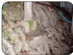
Visible erosion under a deck is common.
